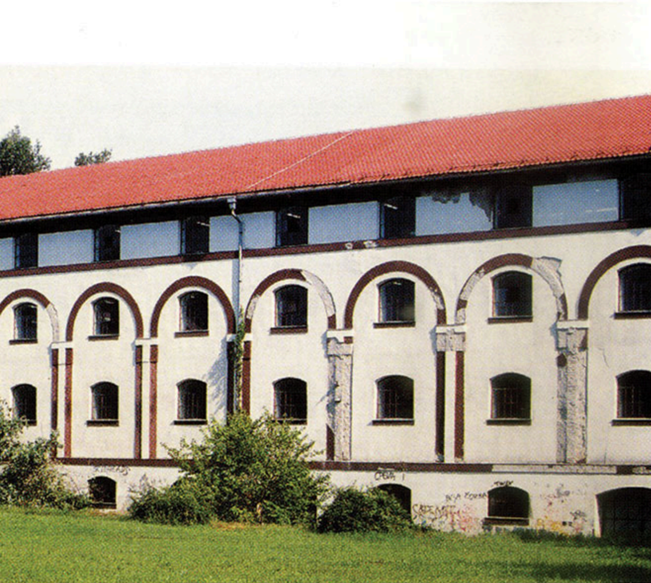
The Matica Srpska Library collections are partially located in the former Czech warehouse built in 1921.
